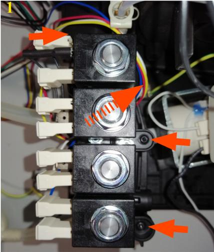
1 Unscrew the screw shown and lift EV assembly
